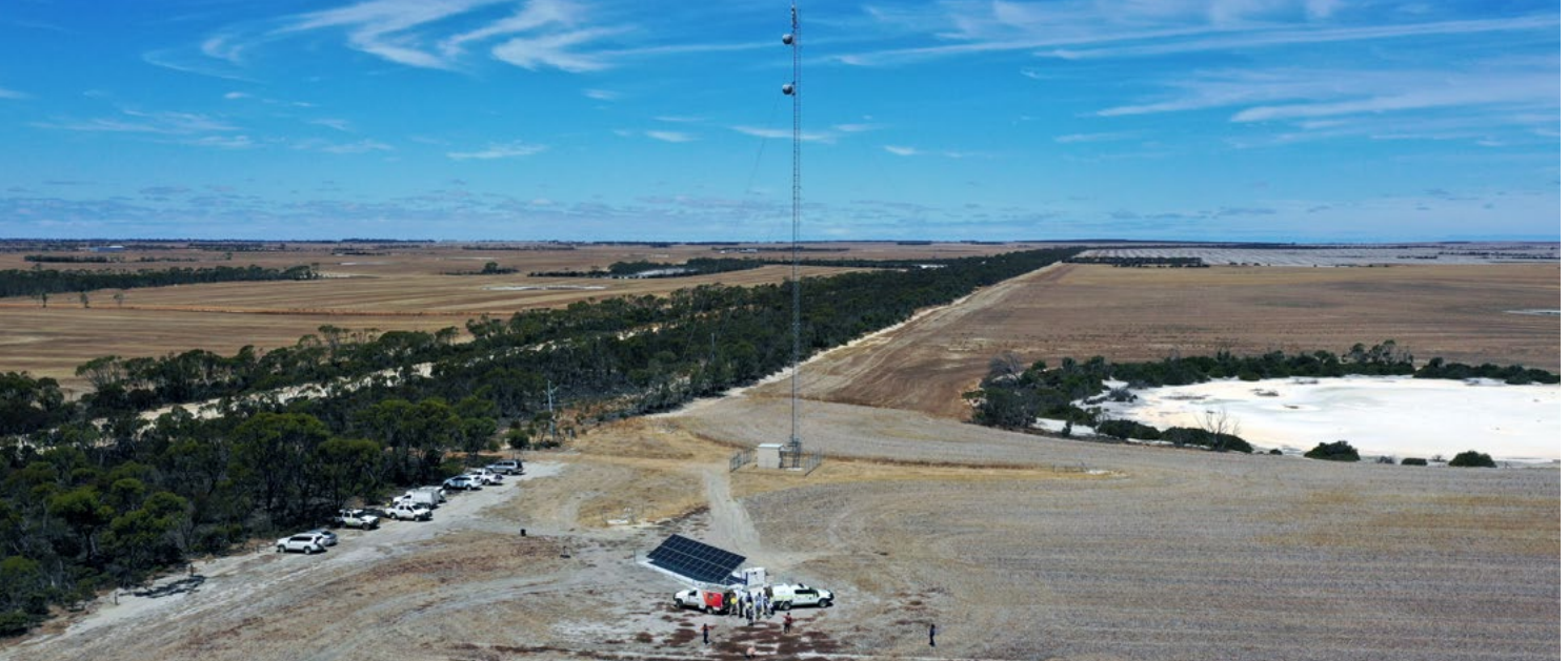
Utility-provided Standalone Power System trial at Mount Ney, Western Australia
